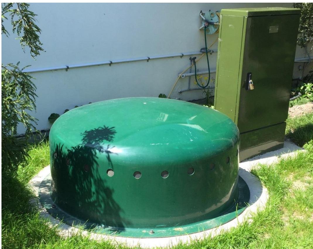
Photo: Settlers Crescent Carbon Filter for PM47 Discharge Odour Control – Station ID OC0501. Includes a 250mm wide concrete ring base pad to give an exposed concrete width of 150 mm.
