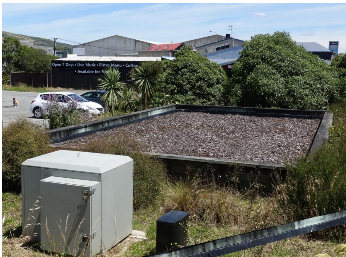
Photo: Ferrymead Biofilter for the PM57 discharge odours. Media almost entirely above ground level with a surrounding timber containment wall. Station ID OC0454.
