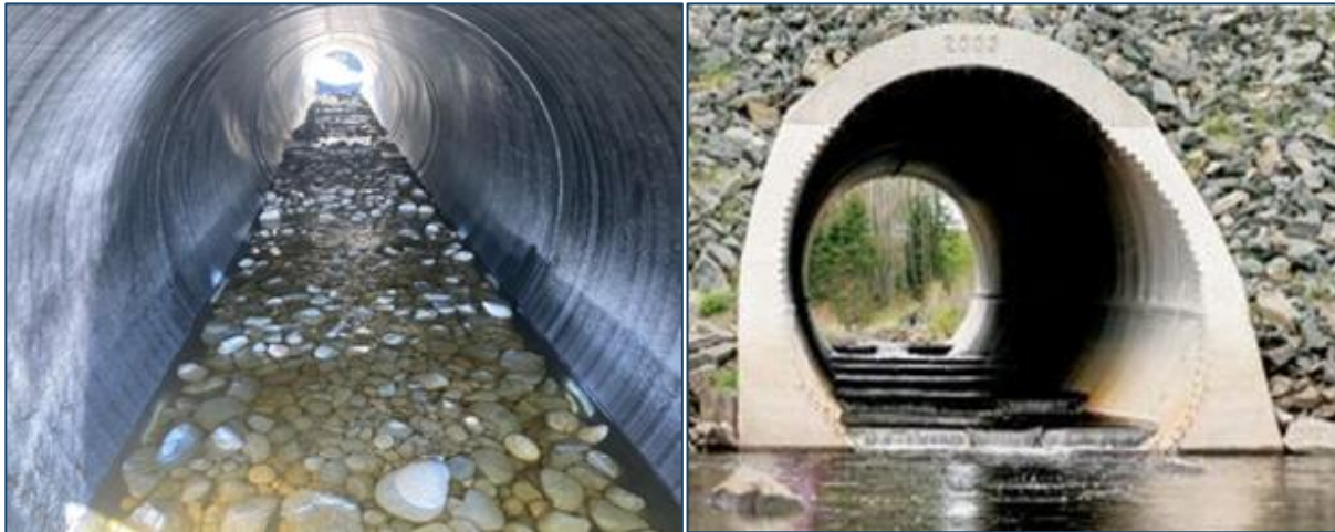
Figure 6: Fish passage examples in culverts
