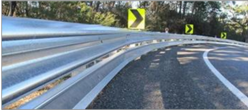
Figure 1: Motorcycle attachment beneath a guardrail
