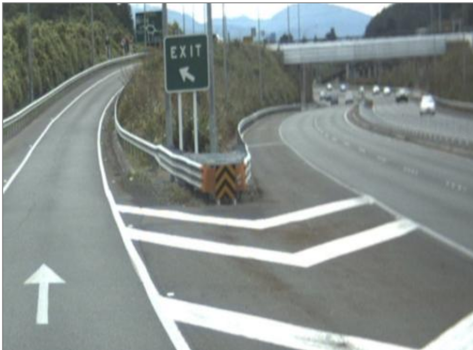
Figure 8: A crash cushion and barriers between two different roads (carriageways)
