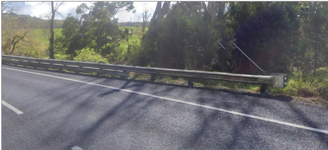
Figure 6: A barrier with a motorcycle attachment
