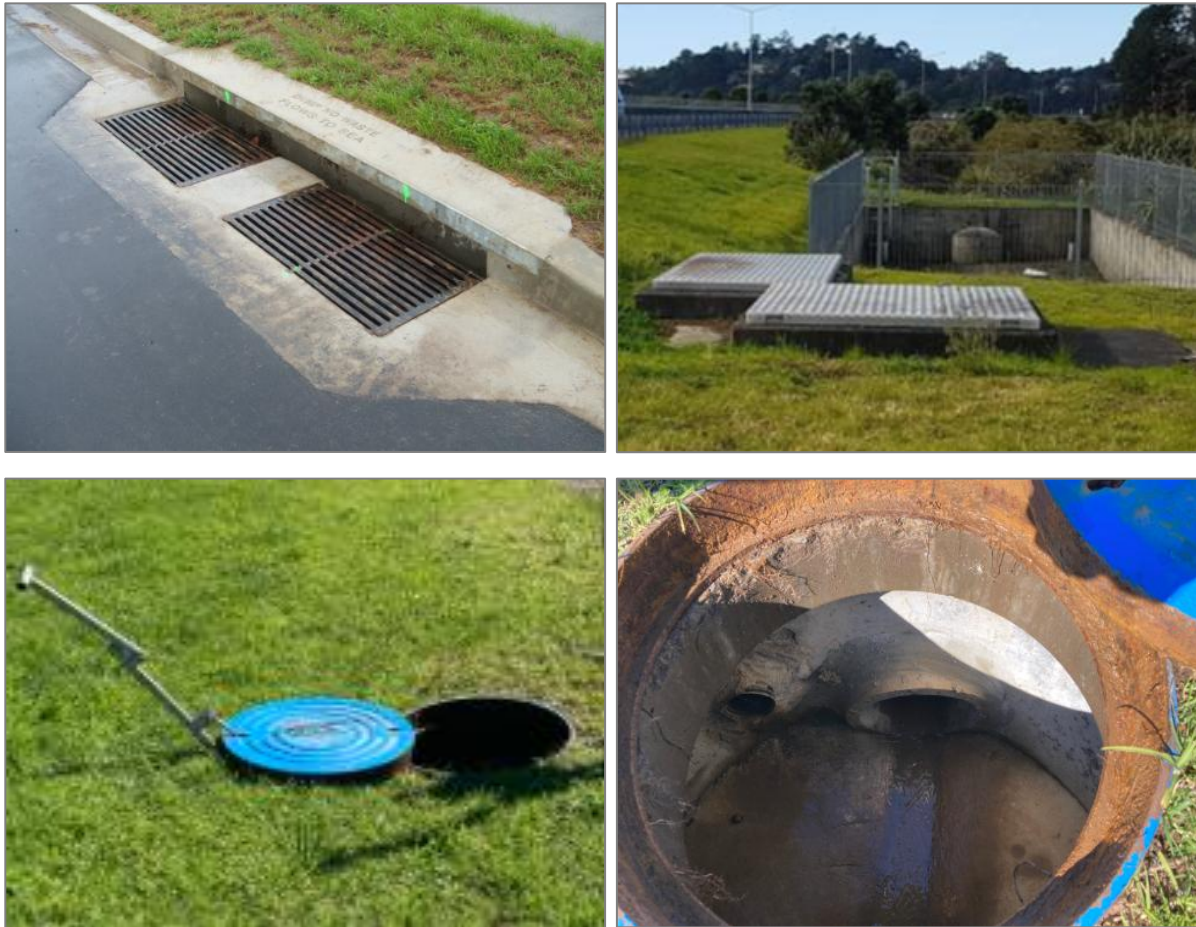
Figure 1: Chamber (drainage) examples
