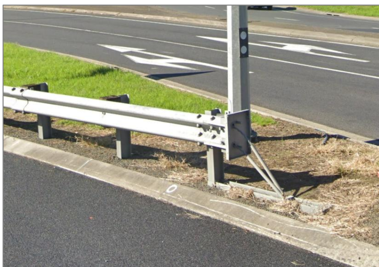
Figure 2: Single barrier with a terminal end
