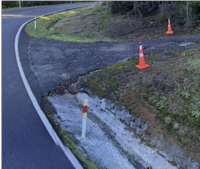
Figure 2: Channels either side of a driveway
