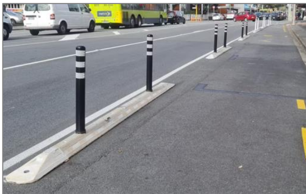
Figure 2: Examples of delineators with a horizontal component (image source https://www.vanguardgroup.co.nz/product/flexible-traffic-separator/ )
