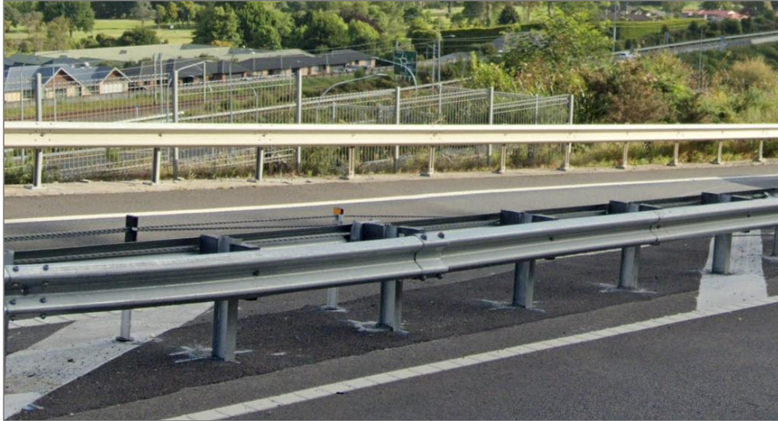
Figure 3: Barrier with rails on both side of the posts
