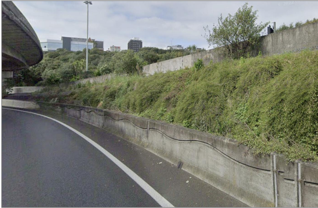
Figure 2: Concrete retaining wall acting as a barrier
