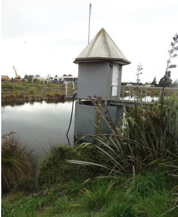
Figure 3 – Octogonal ‘hood’ structure, which house the pump controls
