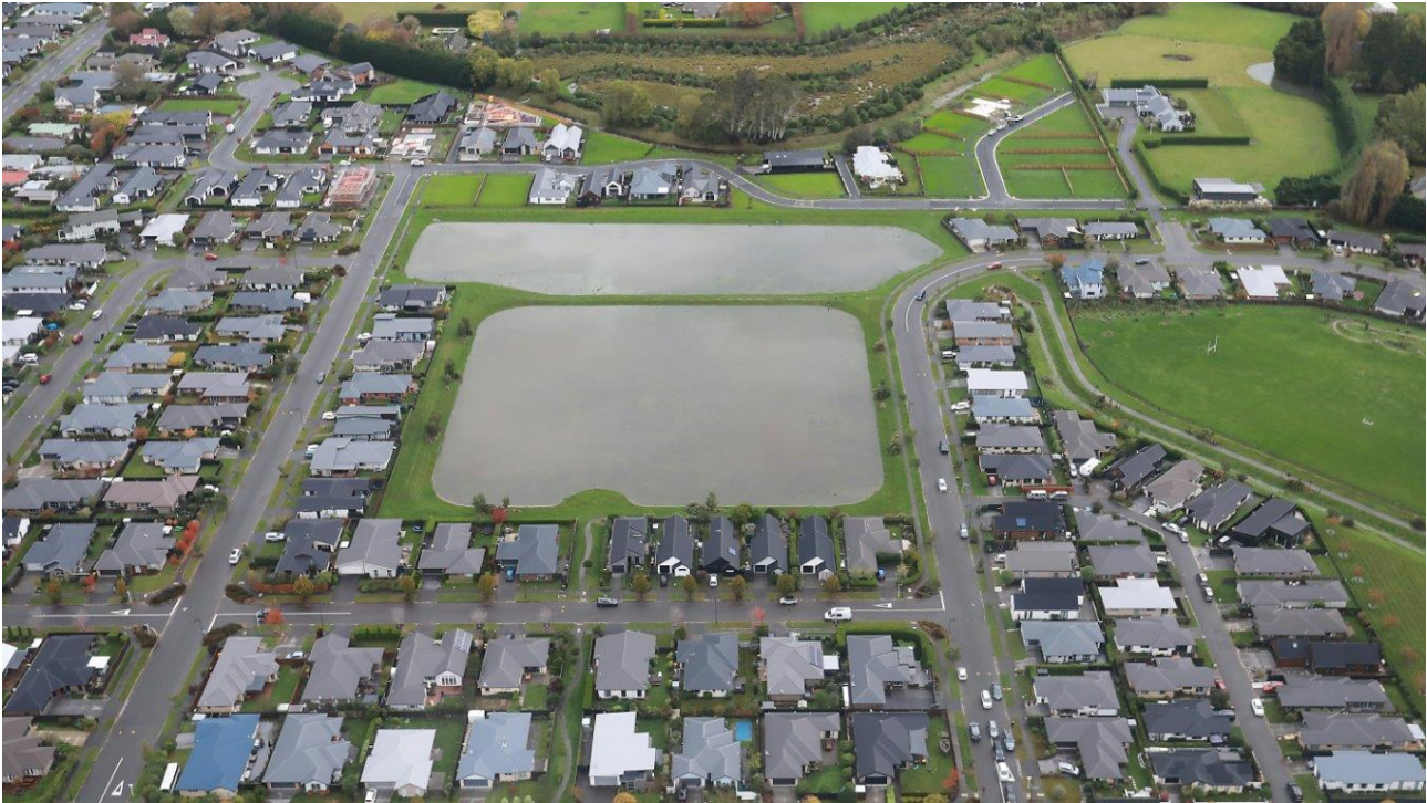
Figure 6-15 Flood photo at Ella Park(Source: ECan). Image source: Map data © 2025 Google
