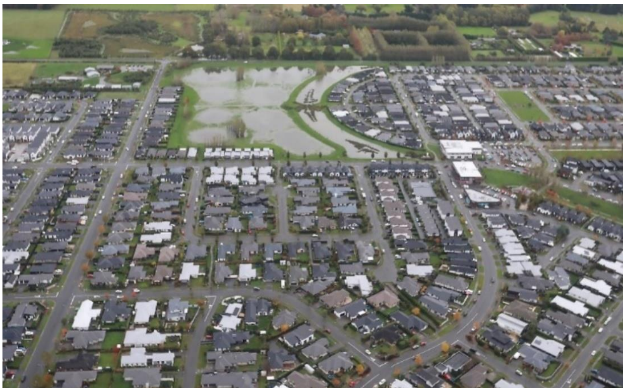
Figure 4-9 Flood photo at Murphys Drainage Reserve (Source:ECan)
