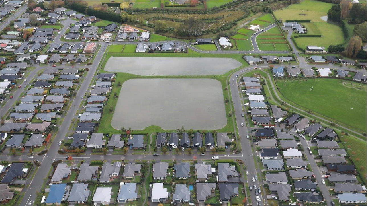
Figure 4-11 Flood photo at Ella Park (Source: ECan)
