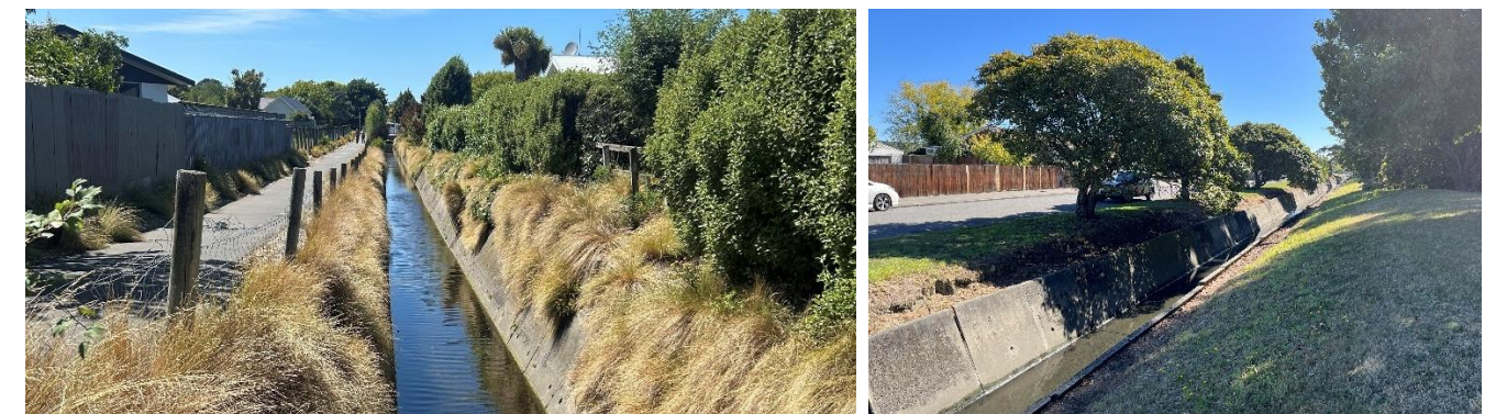
Figure 22: Linwood Canal photos
