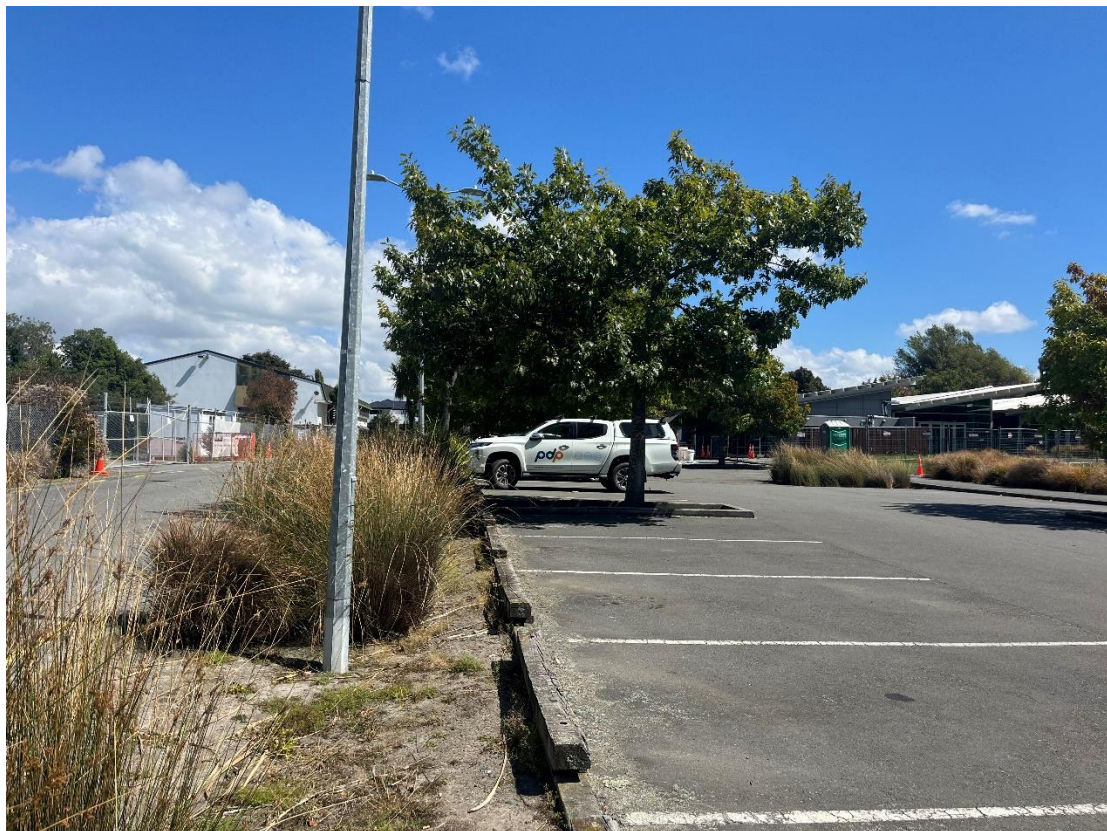
Photograph 6: View of the detention swale at Beckenham Library looking west.
