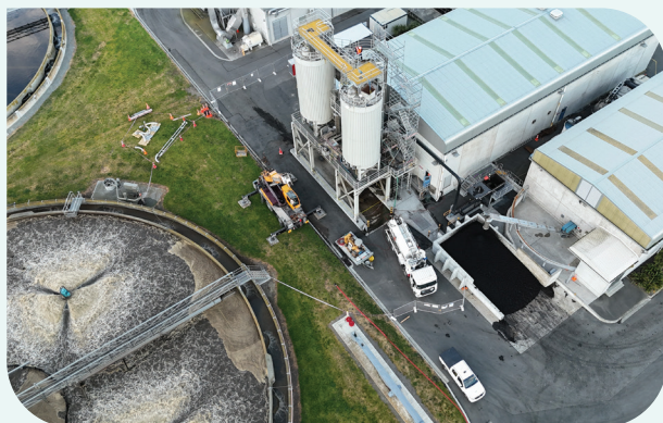
We've been busy carrying out our annual maintenance on the dryers and boilers.
