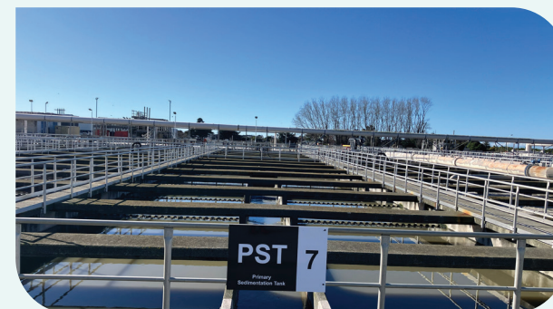
... signage around the plant.
