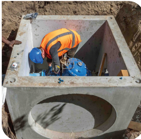
Water pipe work.
