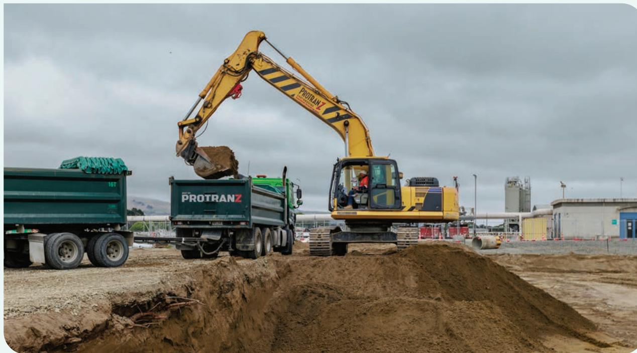
Activated sludge reactor construction charges ahead.
