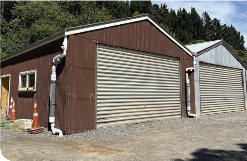
Storminator installed in Akaroa Wastewater Treatment Plant.
