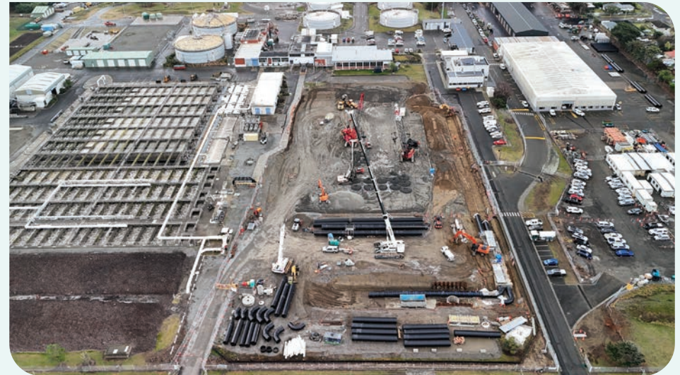
The Christchurch Wastewater Treatment Plant site was busy this quarter
